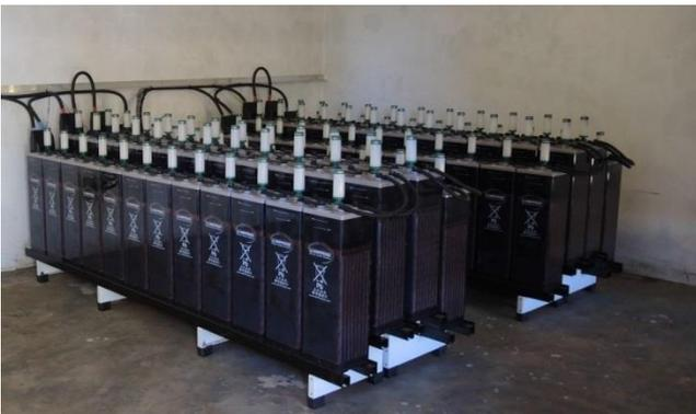
Variations in irradiation and consumption are regulated by the battery, which guarantees a stabile 24 hours power supply system.
